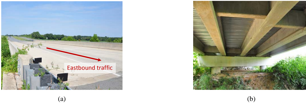
FIGURE 1-2 Bridge photos: (a) top view; (b) bottom view
