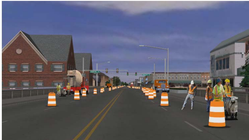
Figure 4-1: Roadway Objects Present in Work Zone
