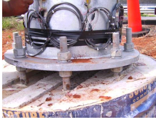
Figure 1.2 Anchor bolts with non-uniform stand-off distances (Fouad et al. 2009)
