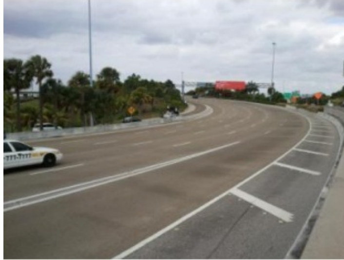
Figure 7-10 Tyregrip HFST System at I-595 Ramp
