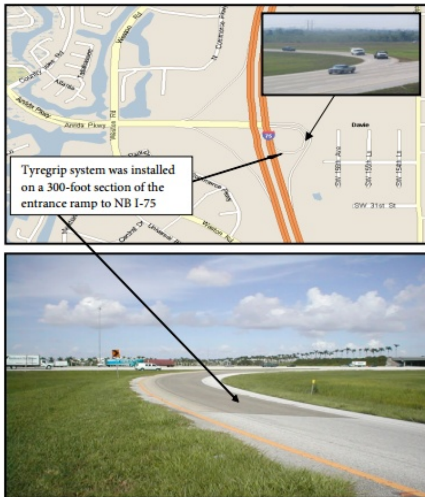
Figure 7-9 Tyregrip HFST System at I-75 Ramp
