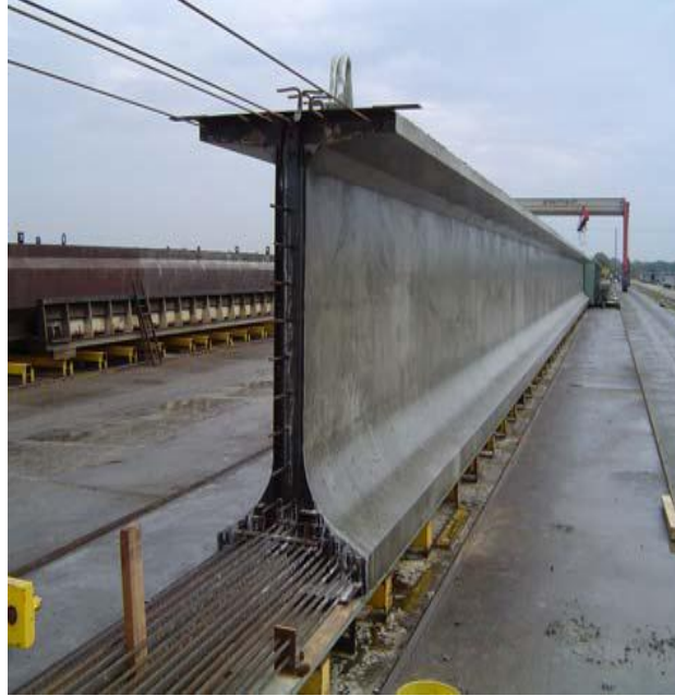
Fig. 7: Florida I-Beam (FIB) Girders under Heavy Vehicle Load
